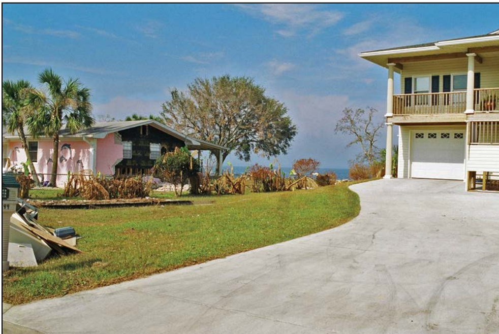
Figure 27: Post-hurricane photo showing an elevated building surrounded by gently sloping fill and an adjacent, damaged, older, non-elevated building
