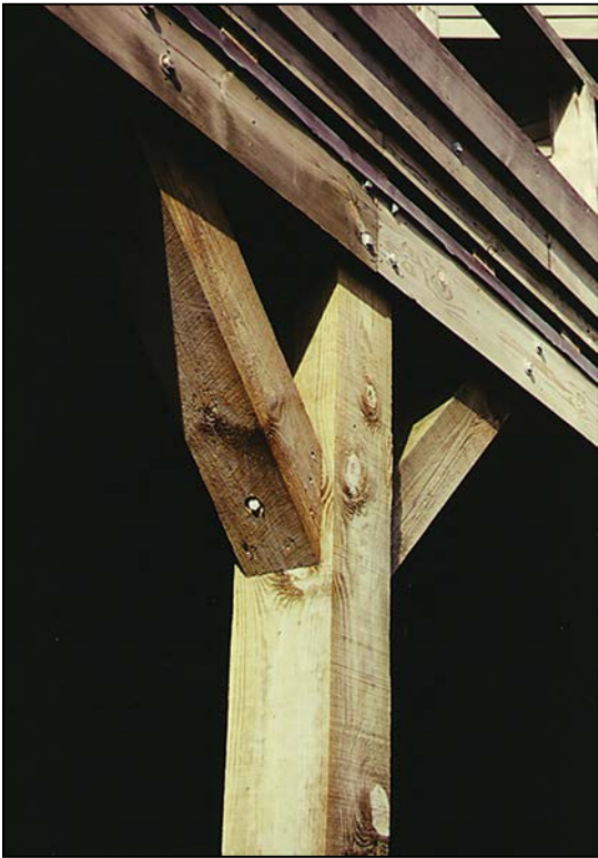
Figure 15: Knee bracing
